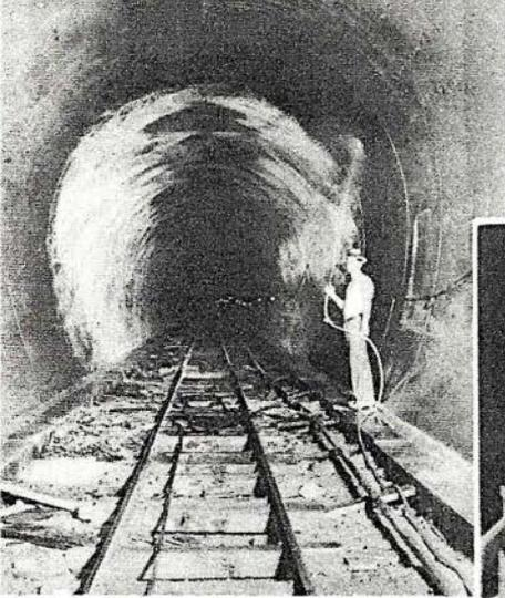
Workman is wetting down finished concrete lining of tunnel to prevent too-rapid drying. This tunnel section is completed.
