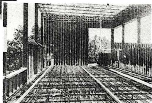
Two-inch layer of beautifully colored concrete is laid over cellular steel framework of ground floor. Hot air passing between steel trusses radiates heat upward through the floor.
