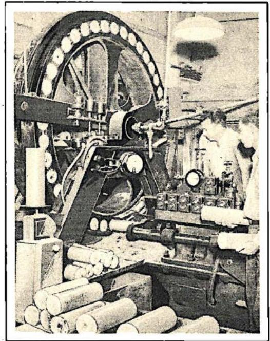
Nine volumes of sawdust are compressed into one log. The logs are forced through the above wheel in firewood lengths.
