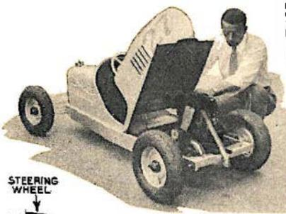
BUILD HOOD OF 22 GAUGE C. R. SHEET METAL, CUT TO WELD ON DOTTED LINE, THEN HAMMER IN THE COWL WITH HAMMER AND BAG OF SHOT
