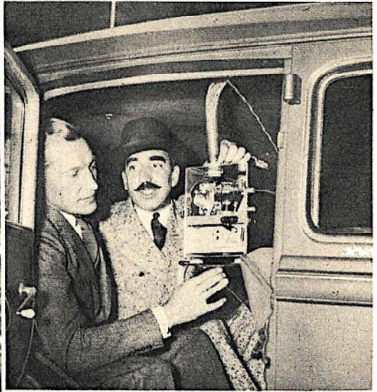
Left—As experimental proof, Lear has mounted his device on an automobile. The loop aerial on the roof picks up the impulses, and the straight aerial in the rear acts as a pointer, to make sure the plane will travel toward rather than away from guiding station. Above—The guiding set is shown installed in auto. It weighs about 30 pounds and is equipped with a dynamotor which supplies power.
