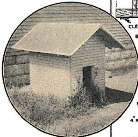
Somewhere around premises can be found a suitable place for a dog house—if you have a dog. This house was made from left-over wainscoting and a bit of roofing paper. Be sure to use false bottom of boards, raised a few inches above ground.
