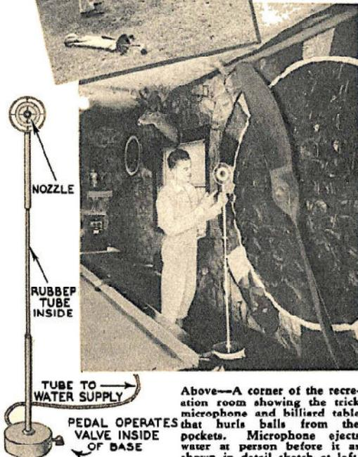
Above—A corner of the recreation room showing the trick microphone and billiard table that hurls balls from the pockets. Microphone ejects water at person before it as shown in detail sketch at left.
