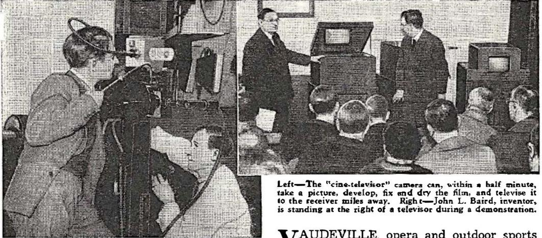
Left—The "cine-televisor" camera can, within a half minute, take a picture, develop, fix and dry the film, and televise it to the receiver miles away. Right—John L. Baird, inventor, is standing at the right of a televisor during a demonstration.
