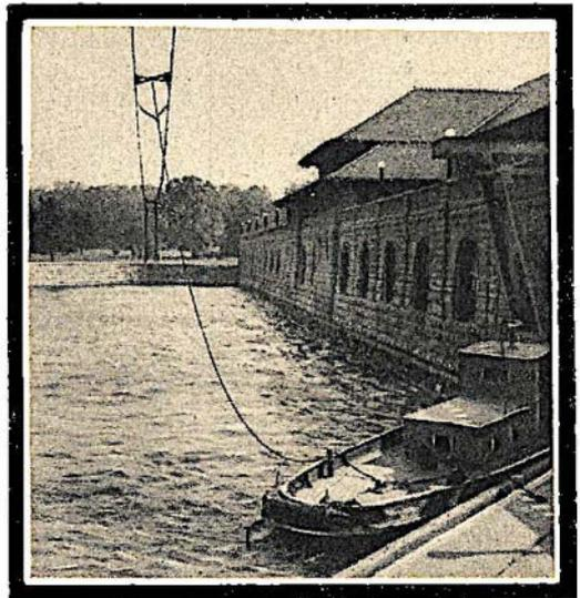
Above boat is powered from an overhead trolley and is used to keep floating refuse from entering power-house turbines.
