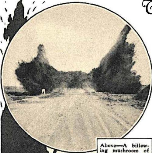
Above—A billowing mushroom of muck shoots skyward as a dynamite blast clears the way through a swamp for a clay and gravel fill. Below—A comparison of Minnesota and New Jersey swamp blasting methods.
