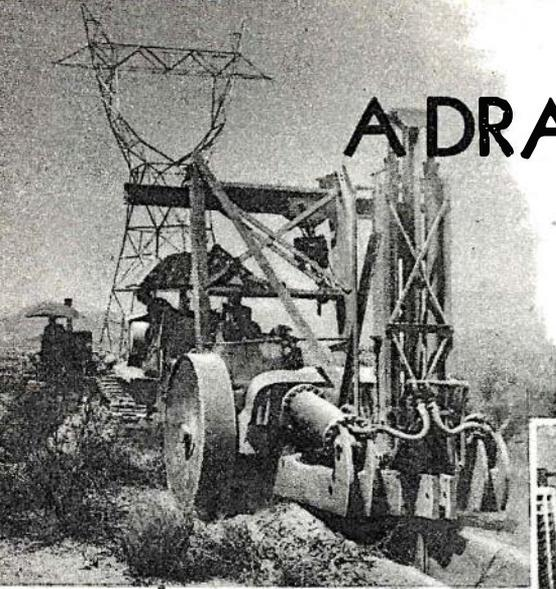
Pulled by caterpillar tractor, this special plow buries counterpoise wire connecting towers in Boulder Dam power line. Plow carries large reel of wire.
