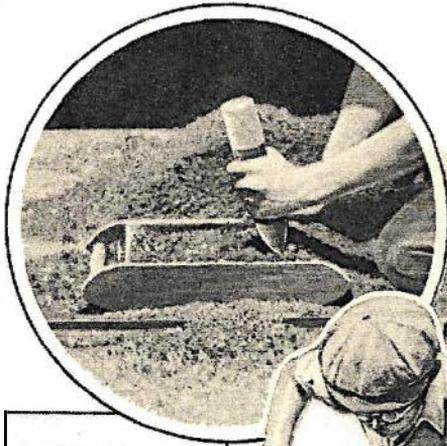
In circle: After pattern is placed, flattest face down, in center of drag, sand is tamped evenly around it, and into every corner of drag. Pack sand just enough so it will stay in place when drag is lifted. Scrape surplus sand off top with any straight bar, then turn over drag and set cope on top. Pack in same way.
