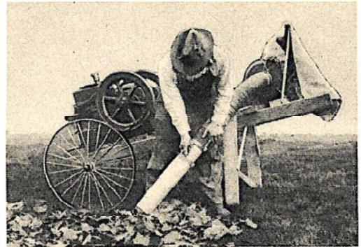
The gasoline motor, set on a two-wheeled truck, sets up a vacuum which draws the leaves up through suction pipe.
