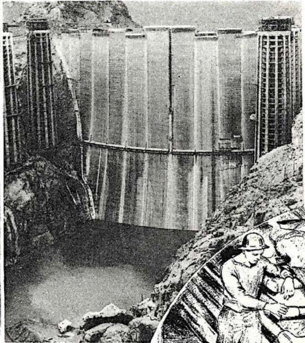
Lowering of this 3,000,000-pound steel door closed first of Colorado river diversion tunnels, marked beginning of huge reservoir which will extend 115 miles upstream, flooding area of 227 square miles. Photo at right shows water level rising behind massive Boulder Dam. Intake towers on either side will eventually be submerged, and then supply water for the power generating plant.
