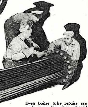
Even boiler tube repairs are made in machine shops aboard ships by Uncle Sam's students.
