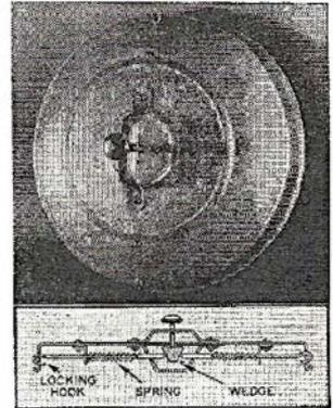
A mechanical lid which will not come off and spill garbage can contents has been devised by a Michigan man. Pressure on a plunger rod passing through the handle and cover releases a spring locking hook which grasps the bead.
