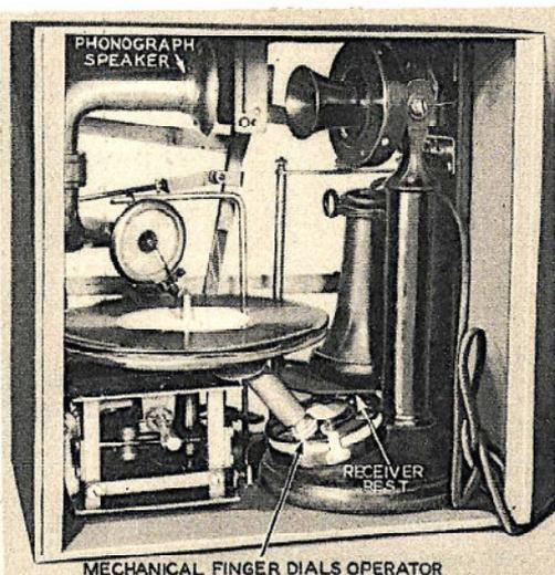
When set off by thermostatic control, this mechanism dials the operator and gives instructions as to location of fire.
