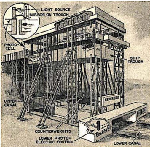
A ray of light, reflected by a mirror into a photo-cell, stops this huge water-filled elevator trough at the canal levels.
