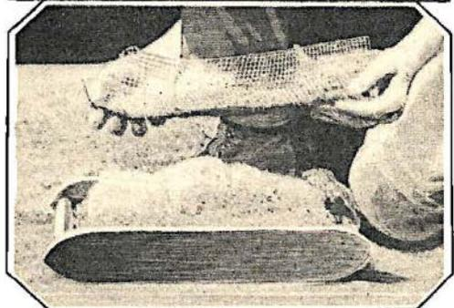
Screen all sand over mold to break up lumps before tamping.
