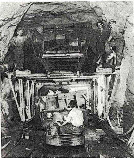
In "grasshopper" method of controlling traffic in tunnels, empty cars are swung overhead while loaded train moves out.
