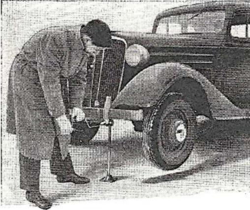
This "standup" jack permits the motorist to lift his car by the back bar of the bumper, without even stooping or soiling his hands. A threaded shaft fits into the removable base and raises the car slowly but safely by crank-spinning.
