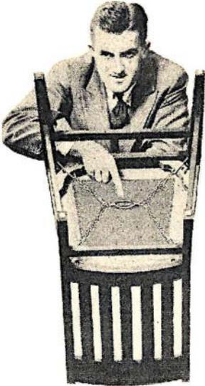
Four hooks are fastened to chair corners and tightened by swivel.
