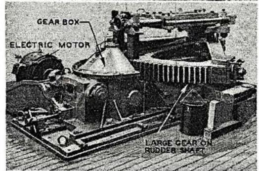
Top: Usual pilot wheel is absent in control room of *Prince Baudoin*, German motor ship. Below—Electric steering device.
