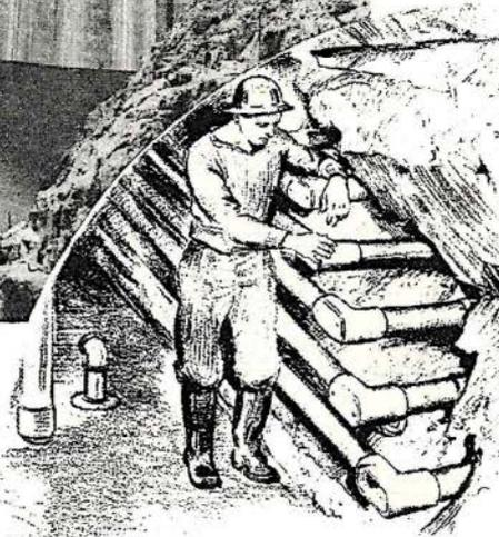
Wires in these pipes lead to 400 thermometers imbedded in concrete of Boulder Dam.
