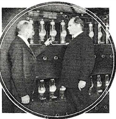
Recent advances in the application of electron tubes have made possible the development of a new type motor. A. H. Mittag and Dr. E. F. W. Alexanderson, consulting engineer, are shown standing before the motor's Thyatron equipment.
