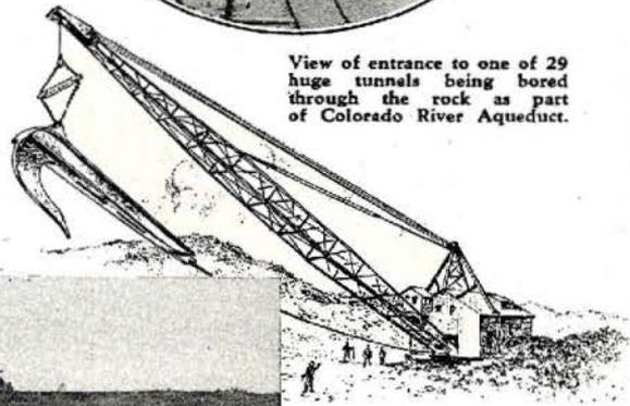
Digging the All-American Canal. When cement, gravel or loose stone is encountered, dragline operator goes fishing with this ten-ton hook to loosen material. Steel line used is two inches thick.
