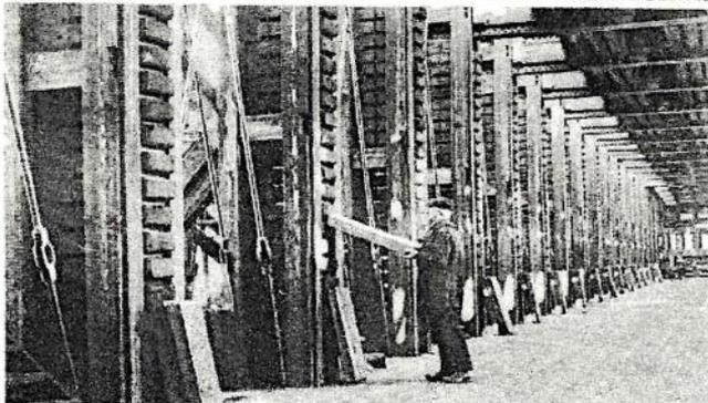
Top photo reveals an oddity in bridges spanning the Mississippi. This unusual bridge can be swung around so allow passage of river boats or closed to permit trains to cross. Lower—Bridge tender removes a wooden plank from one of a long row of rail supports to compensate for rising river.
