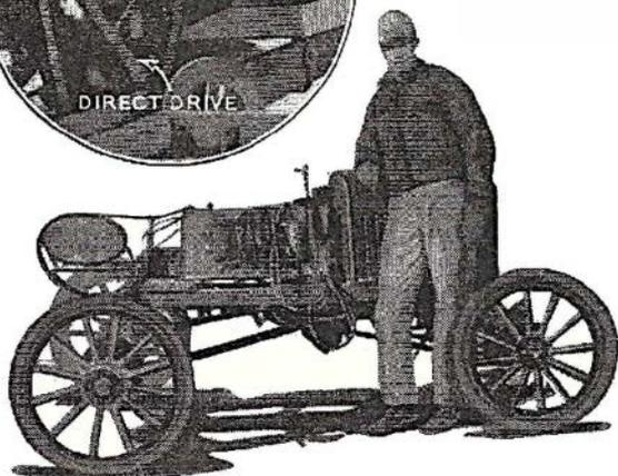
Melvin Johnson built two MM welding generators and mounted them on a shortened Ford. He won first prize of \$5.00. Upper circle shows the two generators. Photo shows Johnson and welding outfit.
